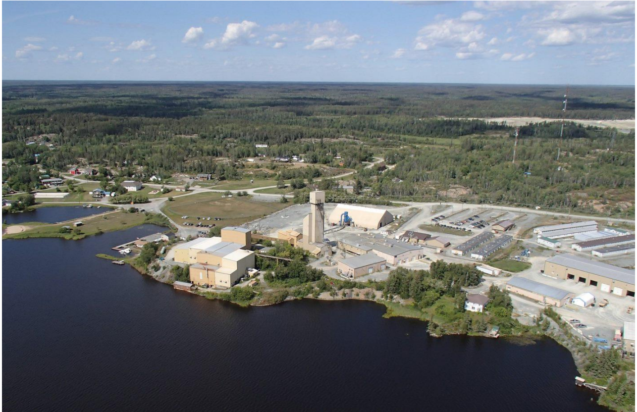
Figure 4: Aerial View Of True North Mill
